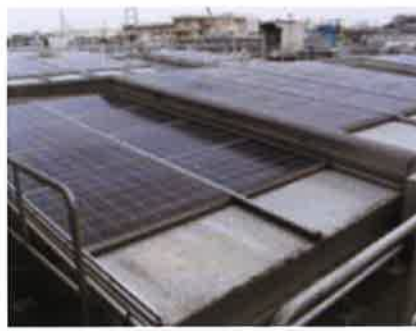
Solar powered system
